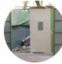
Improper Management of Refuse Collection Point
